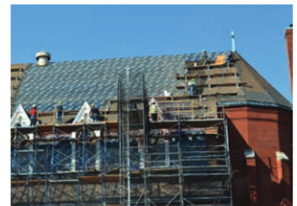
Roof tear-off and dry-in
