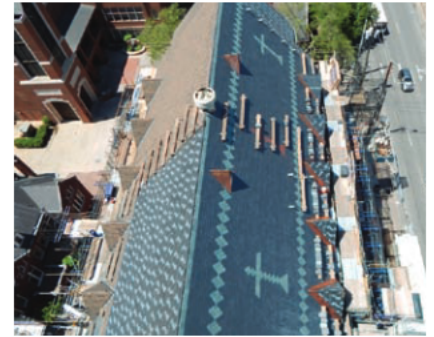
Installing new slate tile
